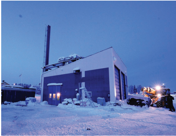
The plant provides all-year-round power for the Hortlax community in northern Sweden
